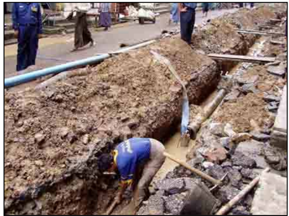
Photo-4 Rehabilitation of old aged pipe
