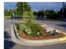
Bioinfiltration in traffic island
