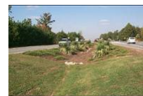
Swale used for roadway drainage
