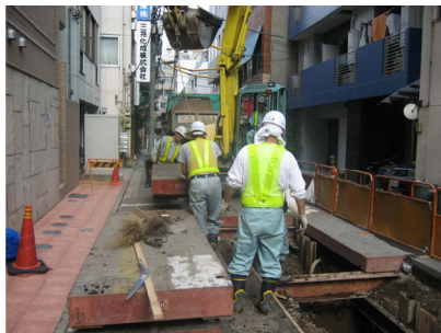
An aged sewer being removed for replacement
