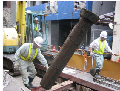
An aged sewer being removed for replacement
