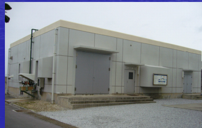
Advanced Wastewater Treatment Plant
