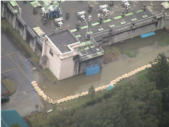
Photo2. A temporary settlement pond and a disinfection plant in Horinouchi Treatment Plant
