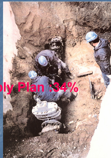
Repairing work of distribution main pipe
