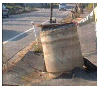
Floating of manhole
