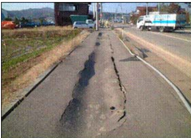
Road surface caving by broken pipe
