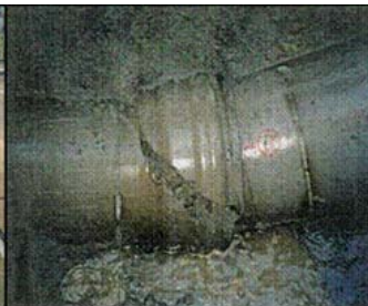
Failure of pipe connection
