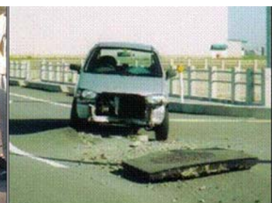
The car which collided with floating manhole
