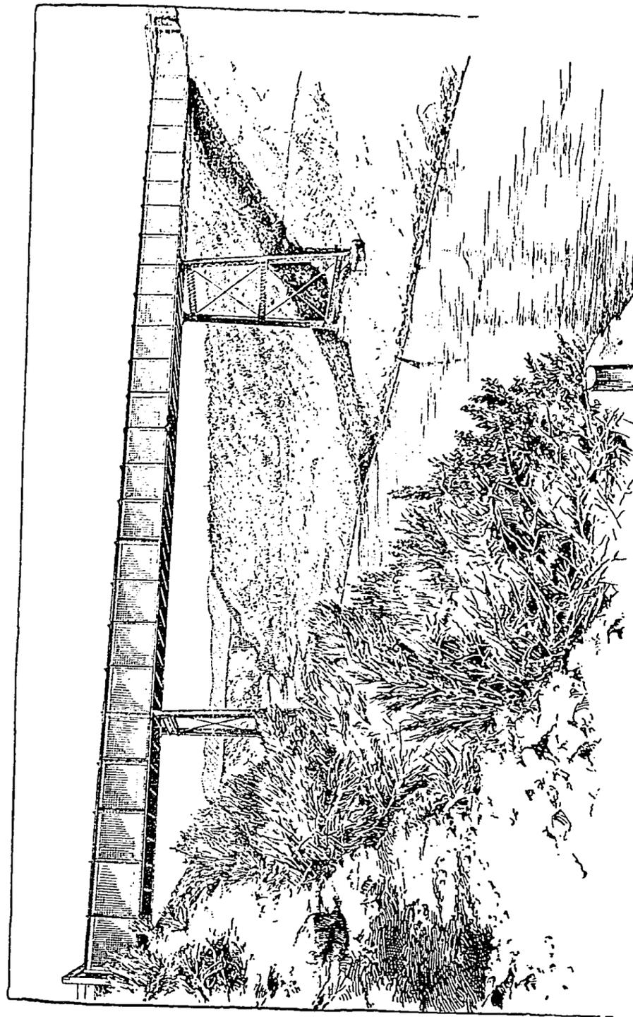
FIG. 30. 130-ft. Plate-girder Flume over Malad River.
