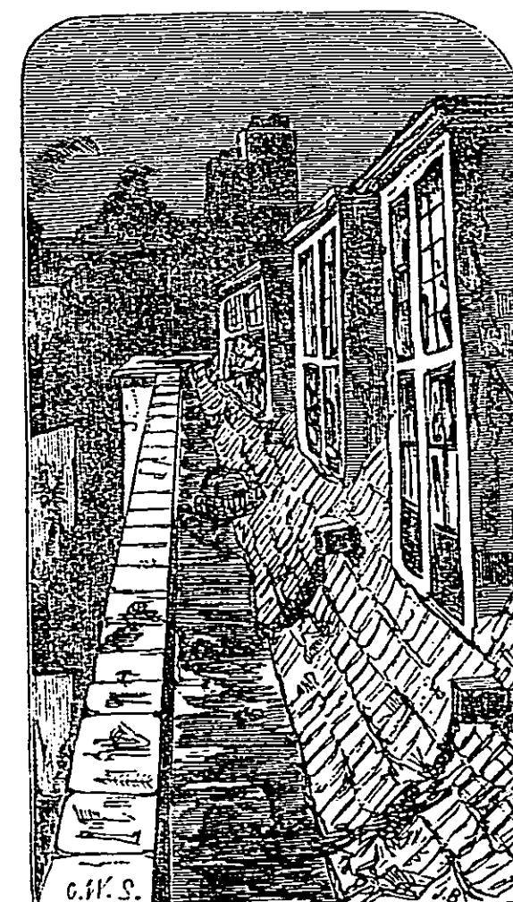
View of the front gutter, as seen from the garret windows.
